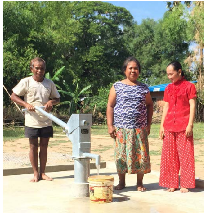
Habitat constructed 24 pump wells in Kouk Reang village to provide families with safe drinking water close to their homes.
