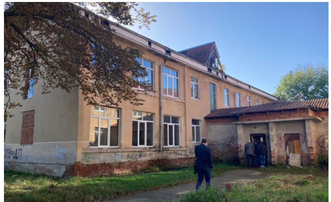
In the city of Kalush at the foothills of the Carpathian Mountains in western Ukraine, the new Habitat branch will transform an abandoned kindergarten into a social housing project that will serve residents in need of a stable place to live.
