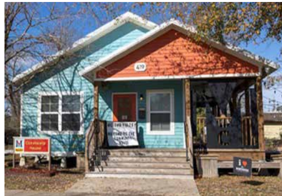
Before Habitat intervened, the McComb-Veazey Community House was in very poor condition. Now, members of the neighborhood feel comfortable meeting in their improved community center.
