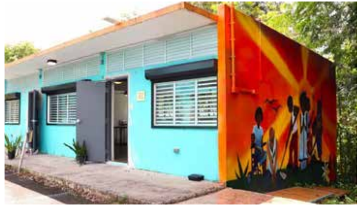
The new energy hub at La Conde helps residents stay connected amid electrical issues and gives them a safe place to shelter during storms.
