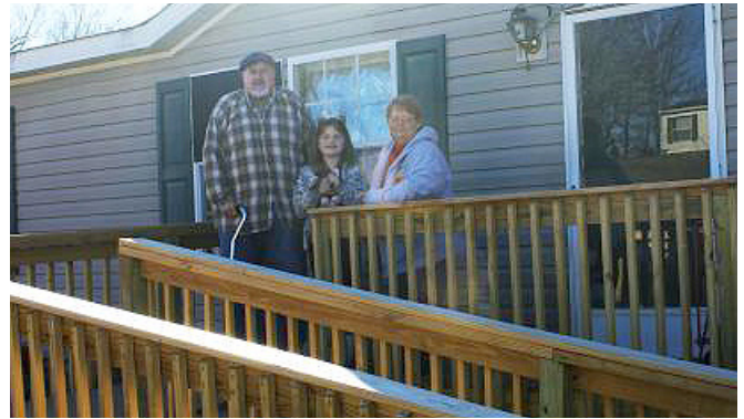
Habitat built a new ramp outside Robert and Teresa's home to ensure they can remain in the home and safely welcome family members.
