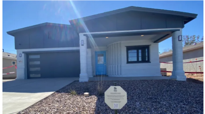
Habitat's first 3D-printed home was built in Tempe, Arizona, from layers of extruded concrete.
